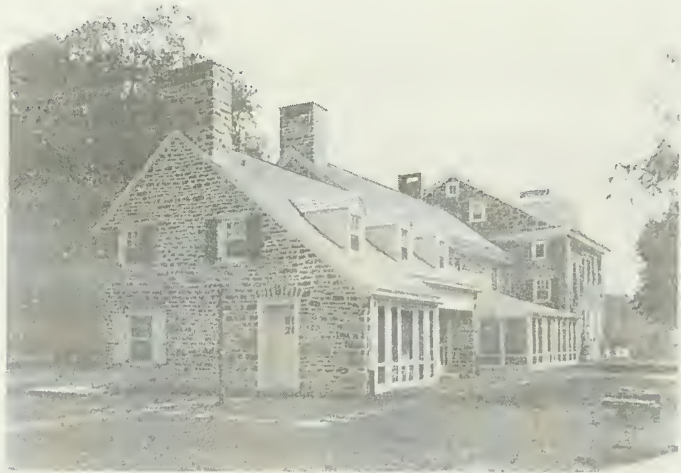
Figure 34 North and West Facades of Manor House, looking southeast, c. 1930
